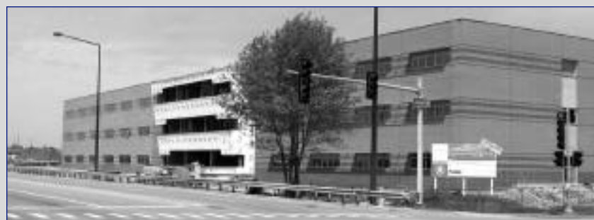
Lower left: Hawthorn's new Townline School will be ready for students this fall.
